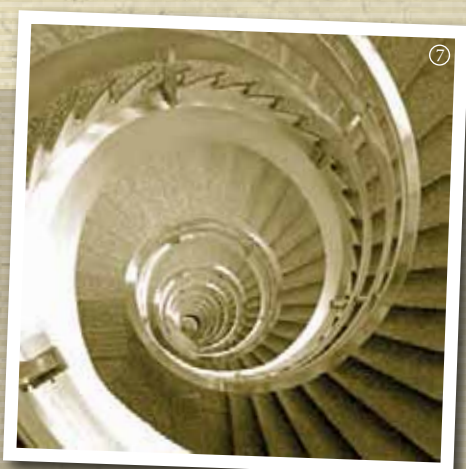
HELICAL STAIRS, ONE OF THE BUILDING'S TRADEMARKS
